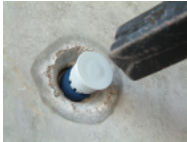
Hammer the Permaseal Form- Tie Plug.
