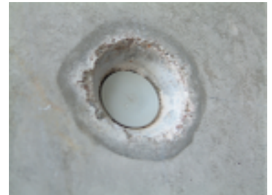
The Permaseal Form Tie Plug installed.
